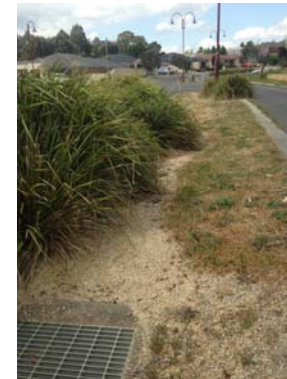
Bioretention swale
